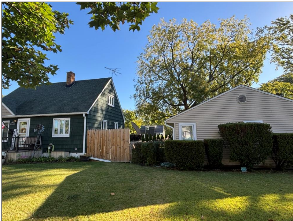
2861 Scott St. – Existing Site looking southerly
