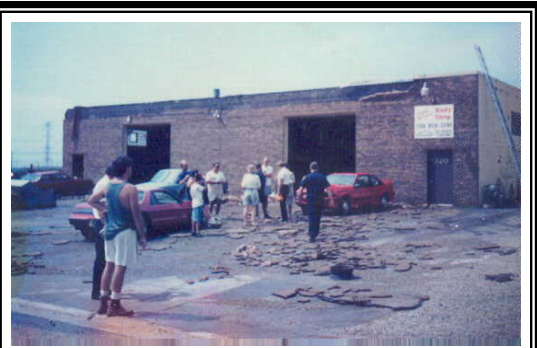
Building damaged by microburst, July 7, 1994 storm in Aurora Aurora Emergency Management
