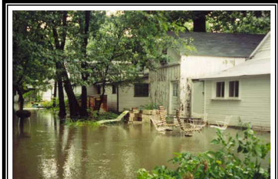
Building flooding in the Methodist Campground
