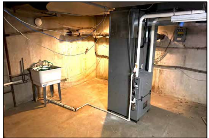
28. Suspect former boiler room inside basement.
