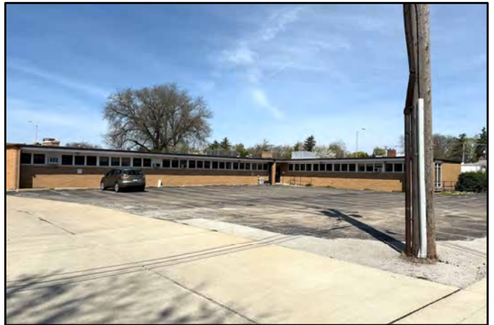
4. Northwesterly view of southeast corner of subject property; observe parking lot off east side of subject building.
