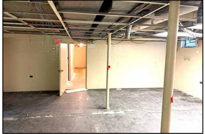
26. Activity room inside basement; observe removed floor tiles.
