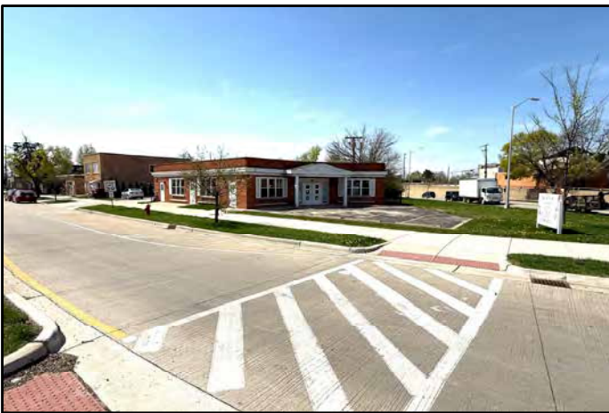
9. Southwesterly view of day care facility on west adjoining property across Broadway Street.
