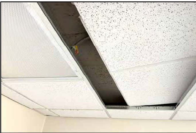
17. 1' x 1' tongue and groove ceiling tiles above 2' x 4' drop ceiling tiles inside subject building; sporadic.
