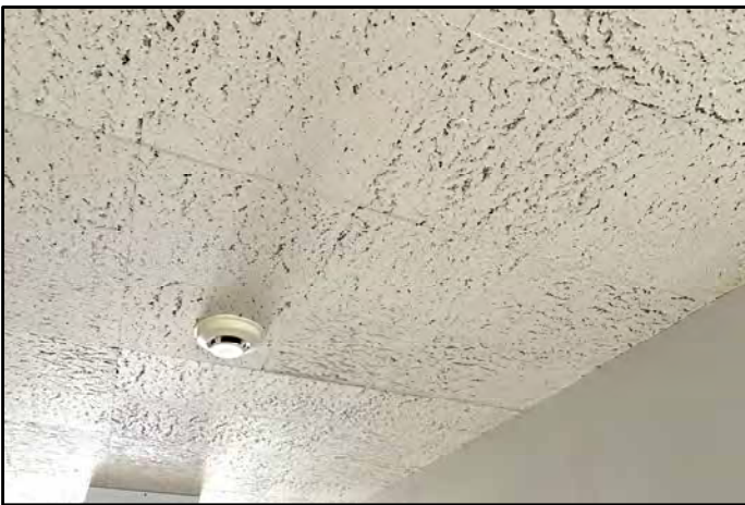
15. 1' x 1' tongue and groove ceiling tiles inside subject building; typical.
