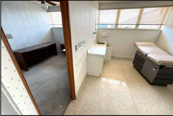
19. Office/examination room inside north end of subject building; typical.
