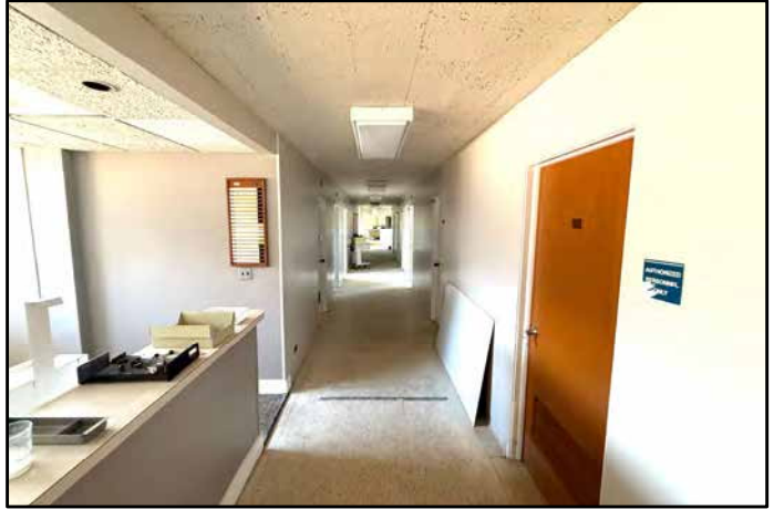
20. North-south hallway inside east end of subject building.
