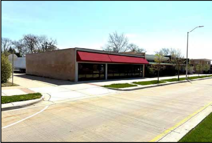
7. Southeasterly view of commercial buildings on south adjoining properties across alley.
