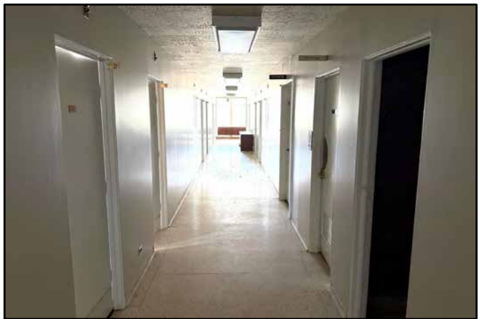
18. East-west hallway inside north end of subject building.
