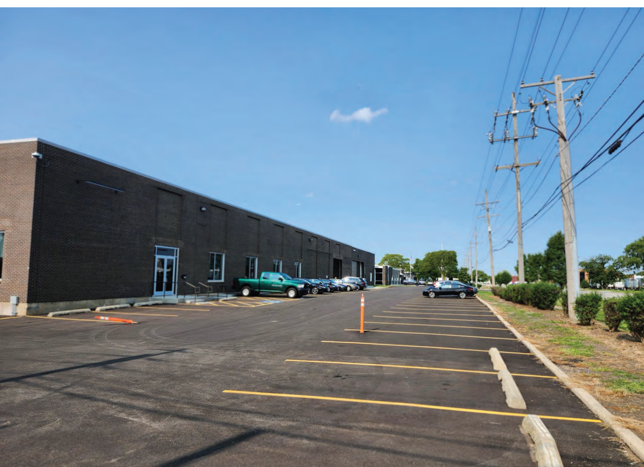
Northeast Corner of Property Facing Southwest
