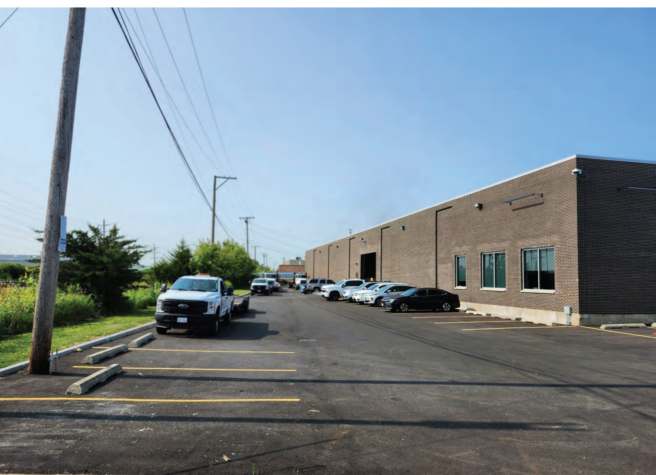
Northeast Corner of Property Facing South
