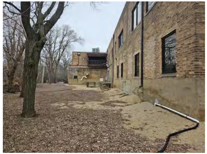
8. East facade, from Northeast corner of building
