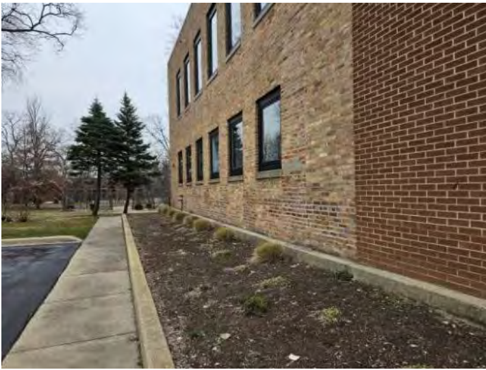
9. West facade from parking lot
