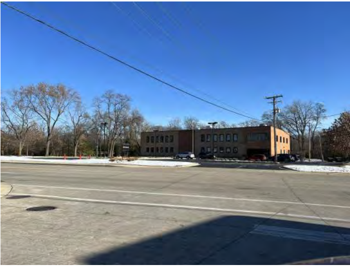
1. West facade from River Rd
