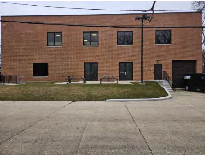
5. South facade from southern paved lot
