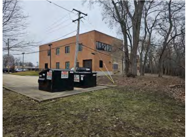
6. Southeast corner of existing building
