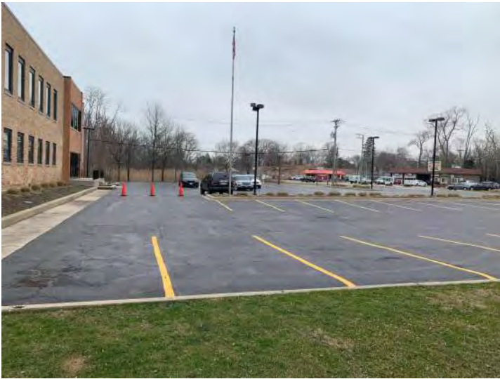
3. View south from north side of exist parking lot
