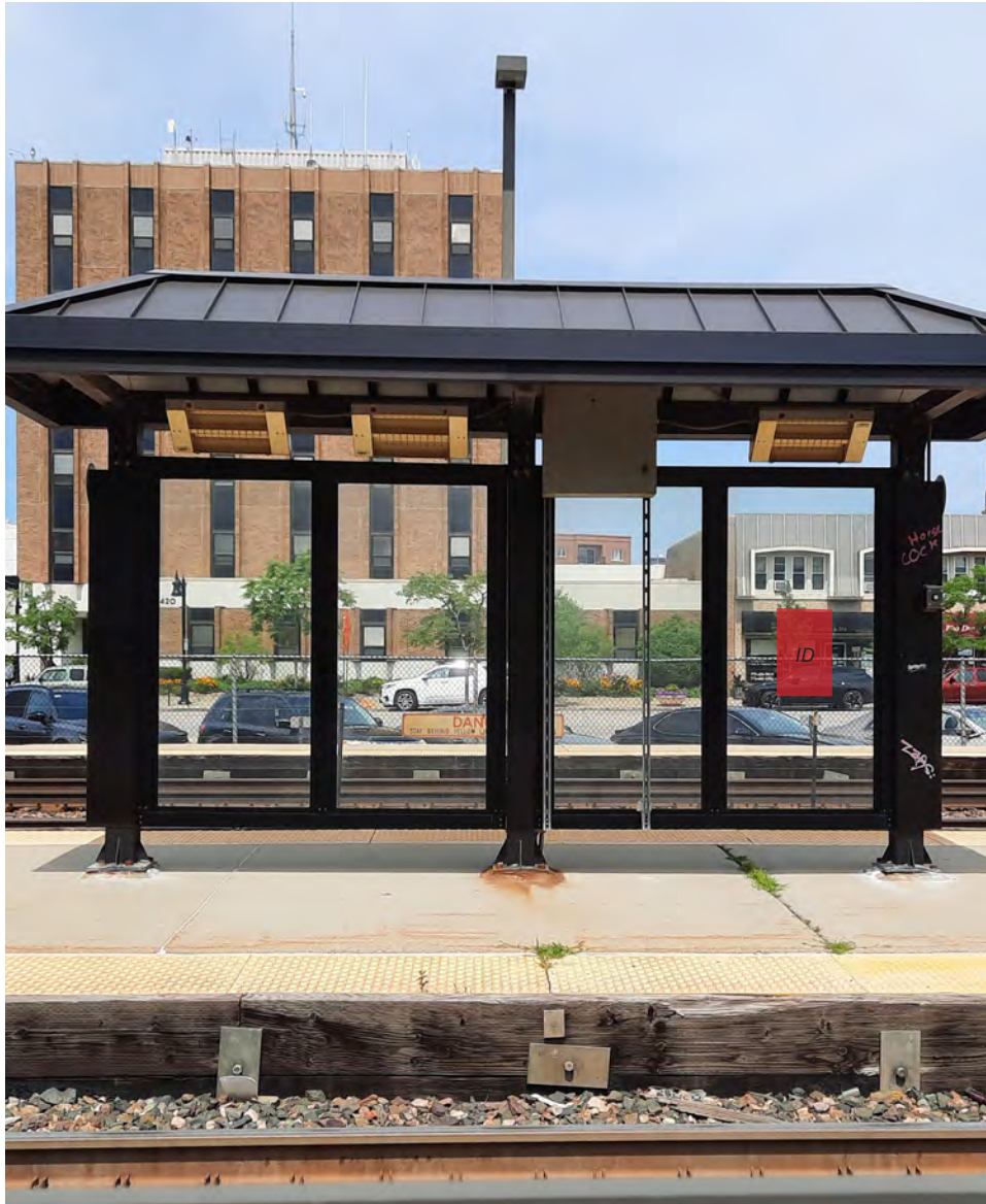
New vinyl graphics installed on shelter window.
