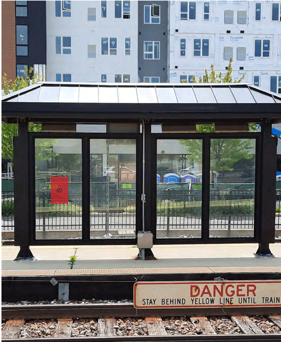
New vinyl graphics installed on shelter window.
