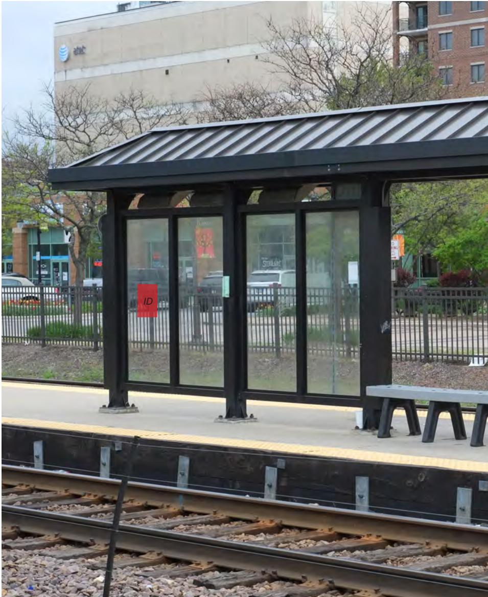
New vinyl graphics installed on shelter window.
