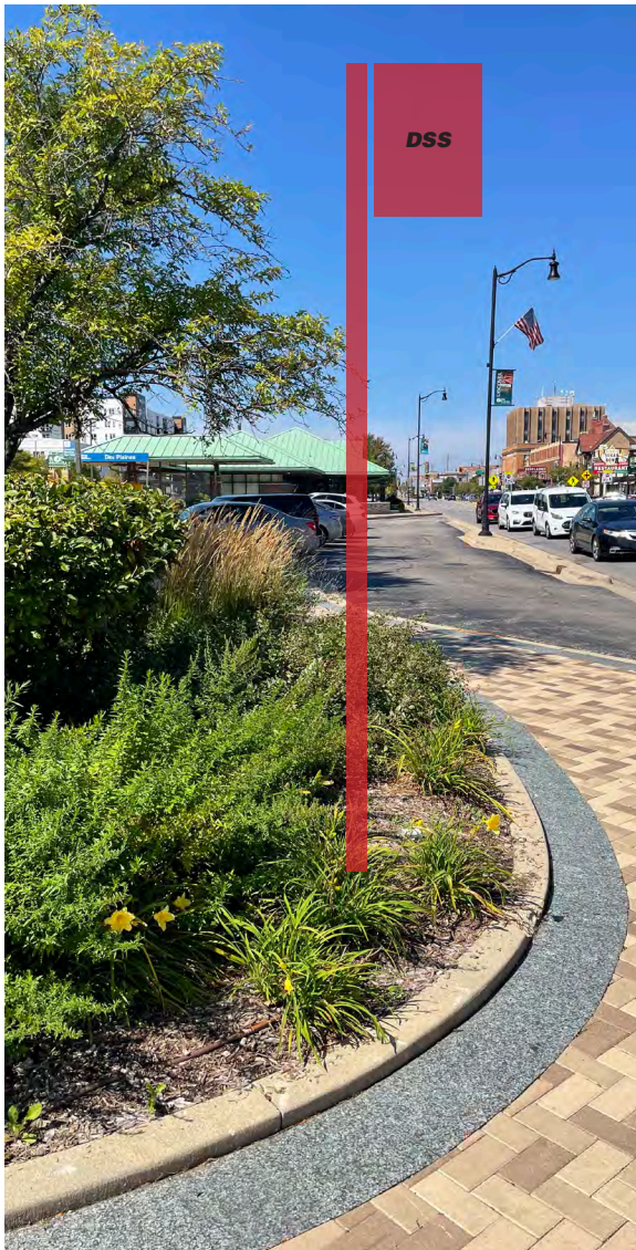
New sign panel mounts to new direct-bury post. Coordinate mounting with DP1-038-N/S (on same bands).
