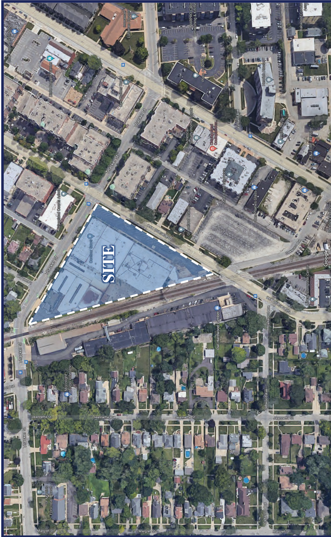
Aerial View of Site
