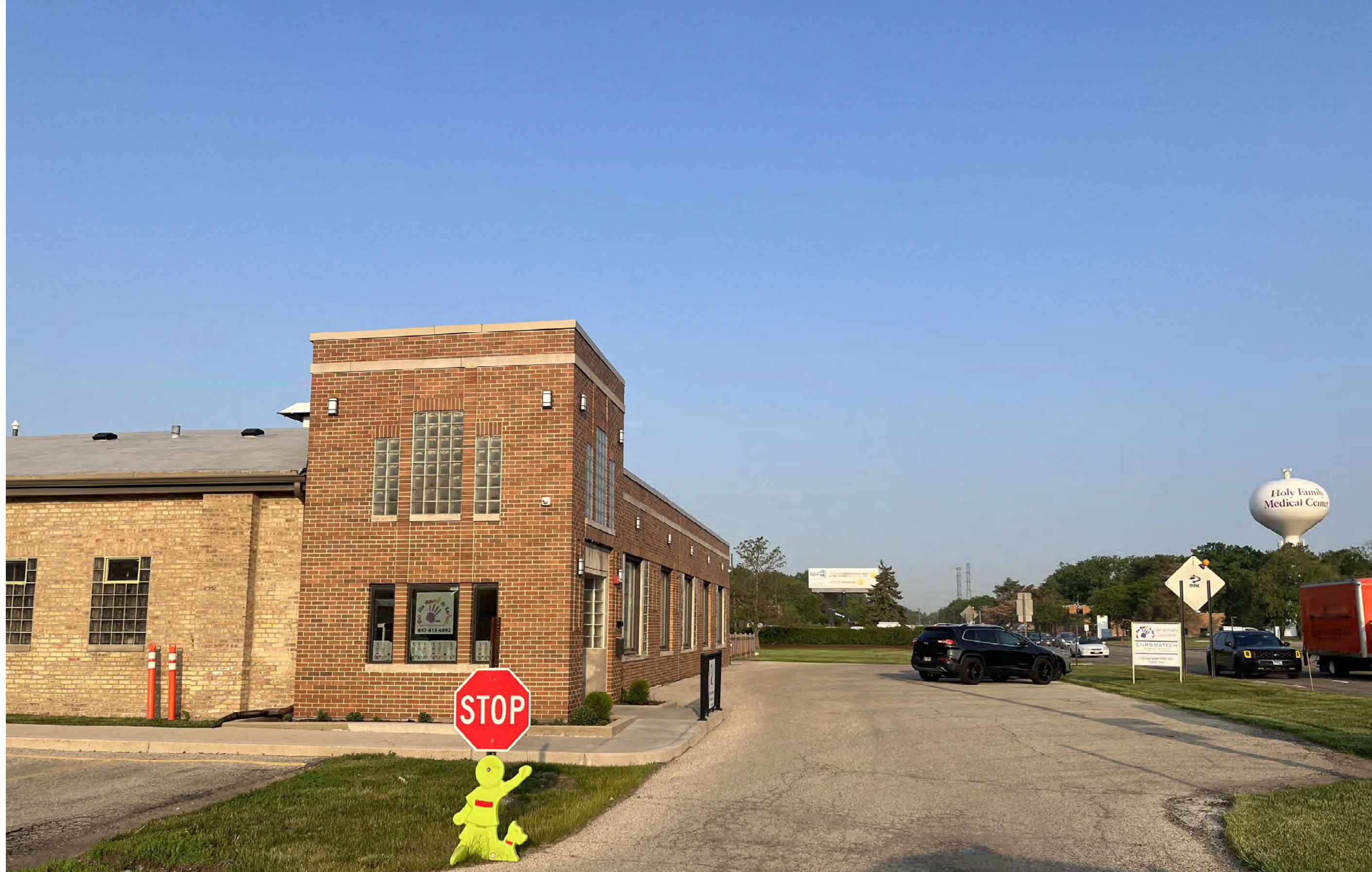
Southeast corner of 1345 E. Golf Road
