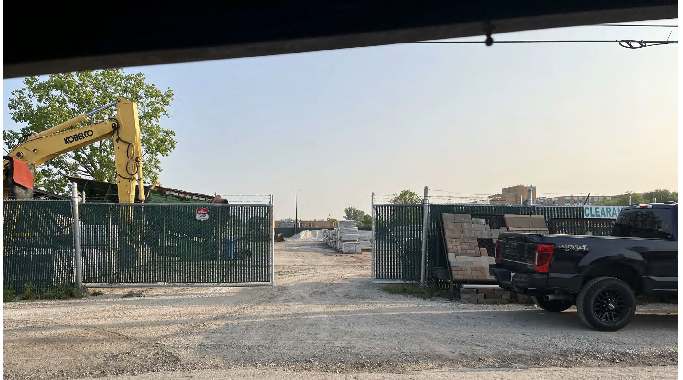
1331 E. Golf looking North (from rear of property)
