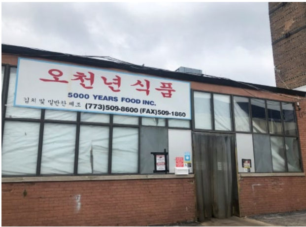
Image 1: Photo of Exterior of Building
