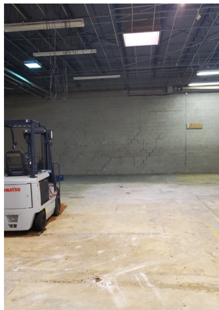
View of inside of building, cleared of debris
