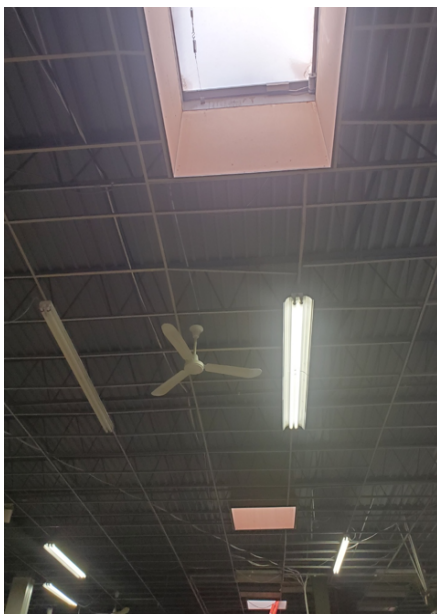
Roof repairs status in June 2023
