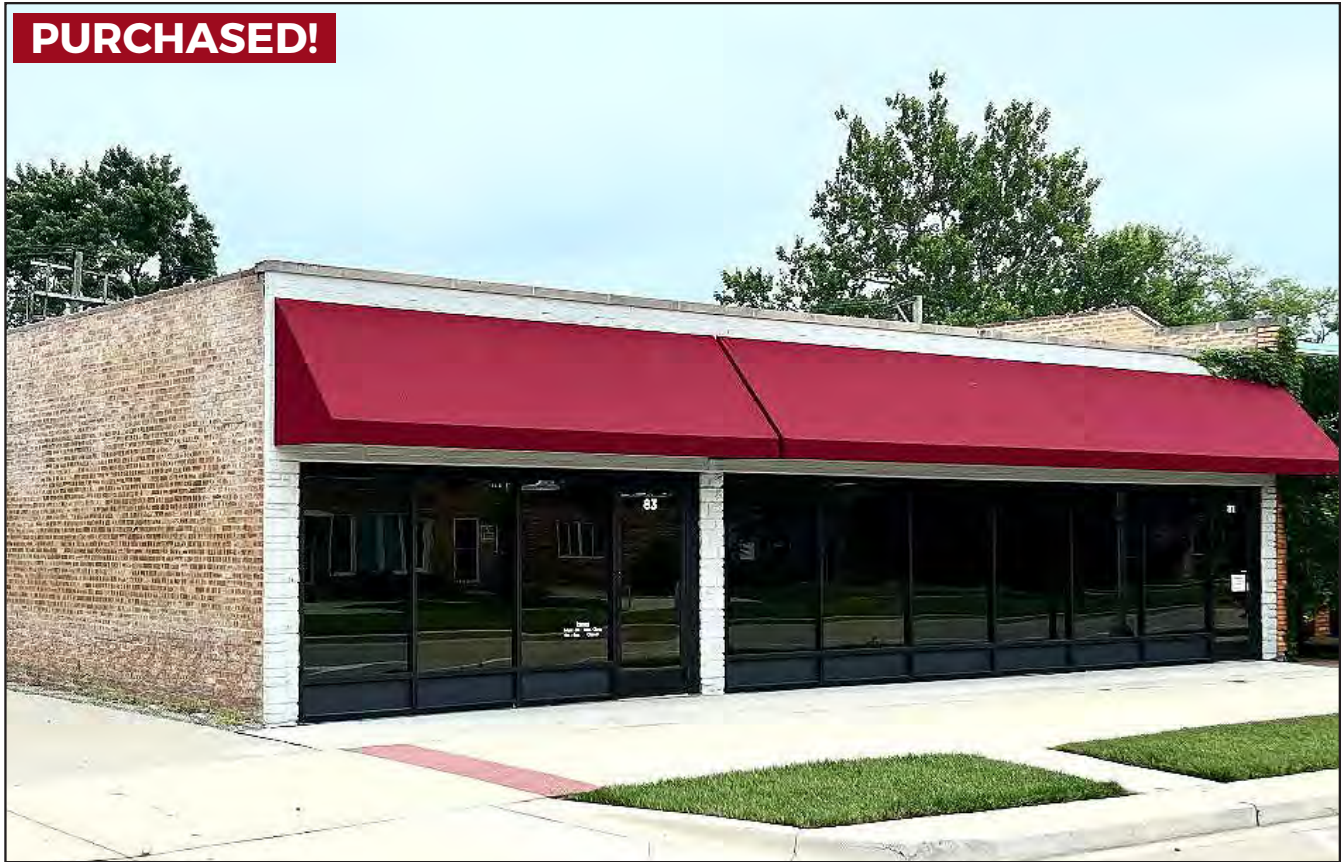
Broadway Street and the Golf Rd. round-about circular intersection have been completely rebuilt in 2019, thus all the new roads and new sidewalks are providing Broadway Street an inviting curb appeal.
