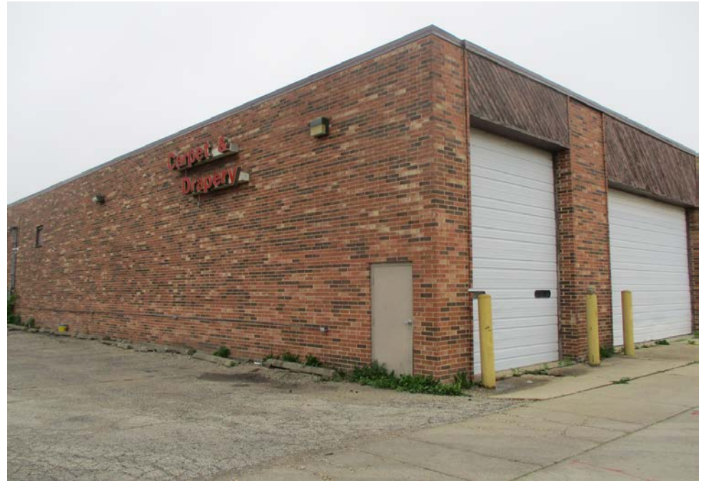
Loading doors along Oakwood Avenue and parking space along alley
