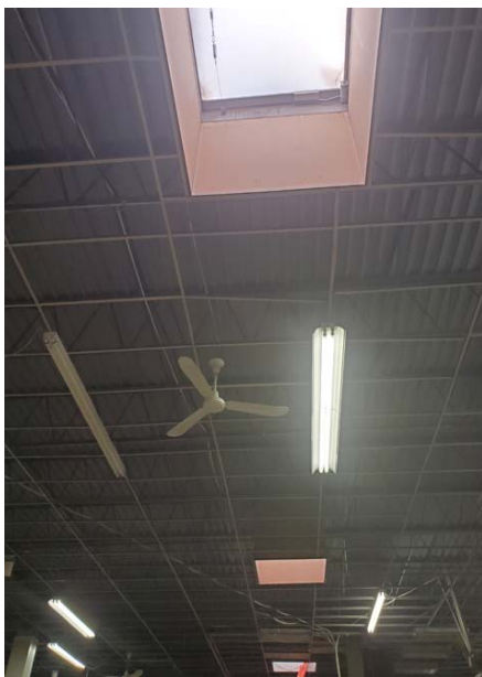
Roof repairs status in June 2023
