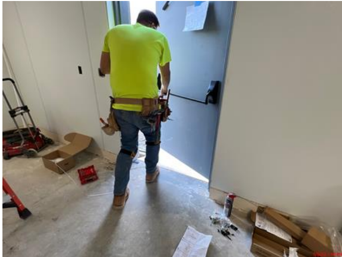
Door hardware being installed.
