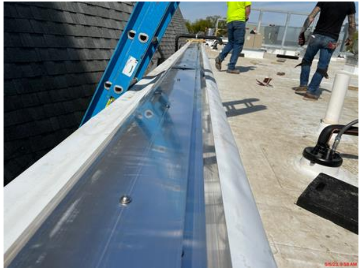
Expansion joint installed.
