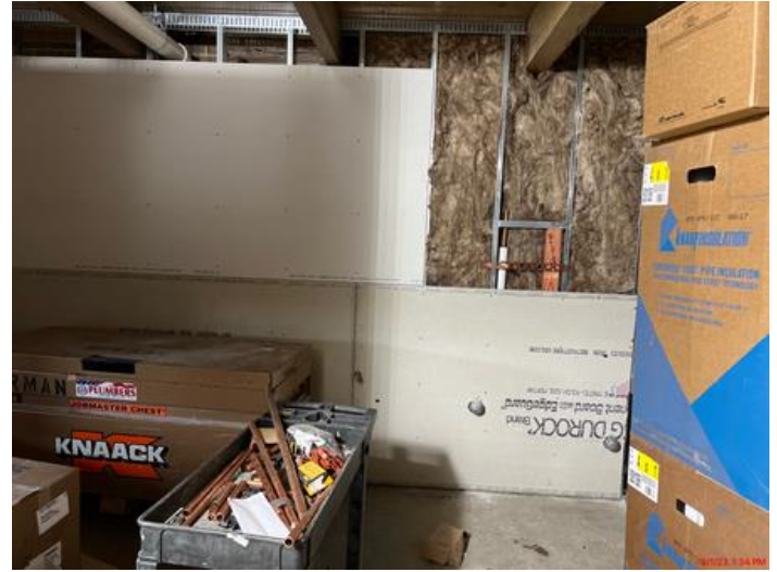
Durock and drywall installed in restrooms.
