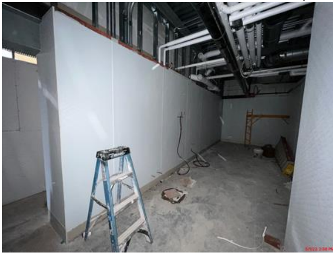
FRP done being installed in kitchen.
