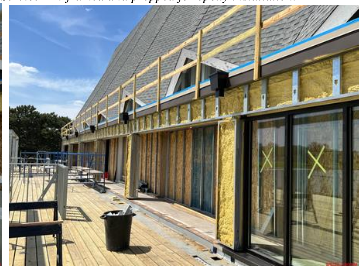
South elevation exterior wall framed.
