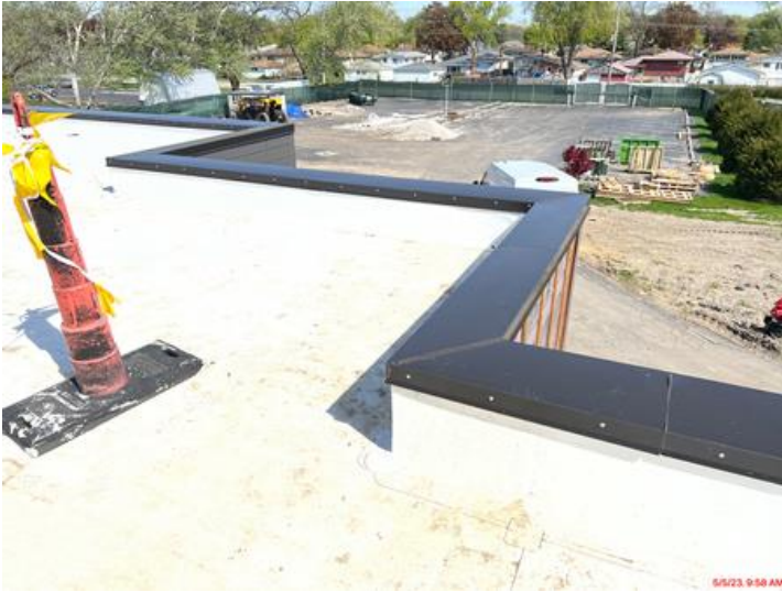
Break metal installed at parapet wall.
