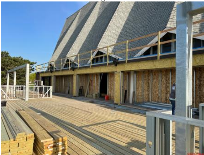
South elevation exterior wall framed.
