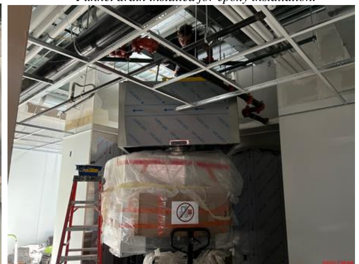
Black iron being installed over pizza oven.
