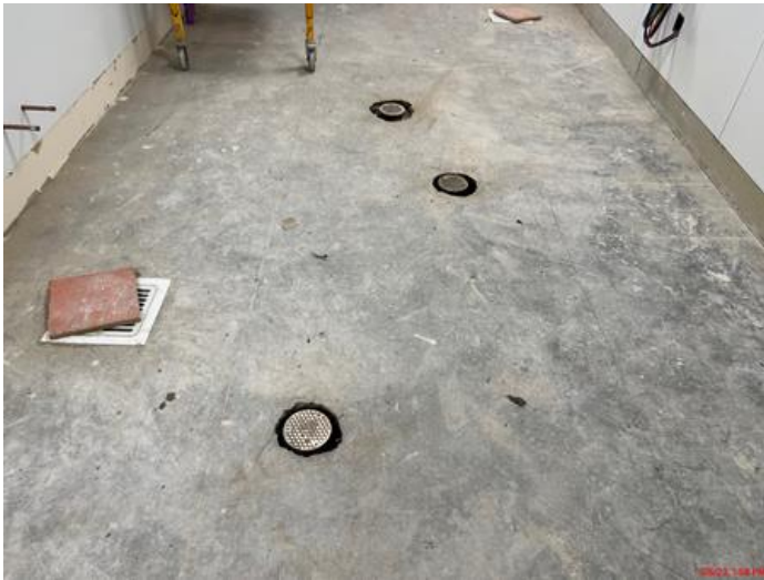
Drains exposed for epoxy installation Monday.
