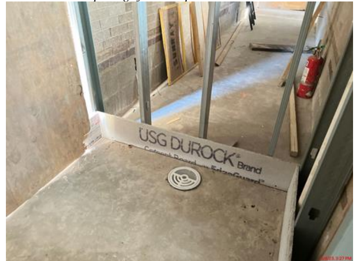
Service 116 framed and prepped for epoxy installation.
