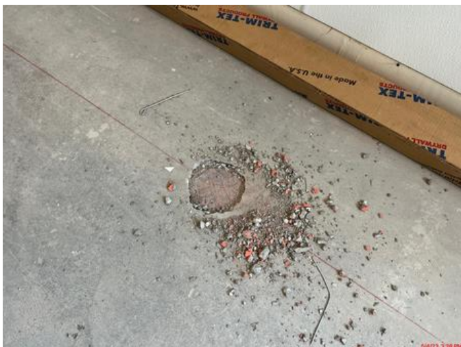
Drains exposed for epoxy installation Monday.
