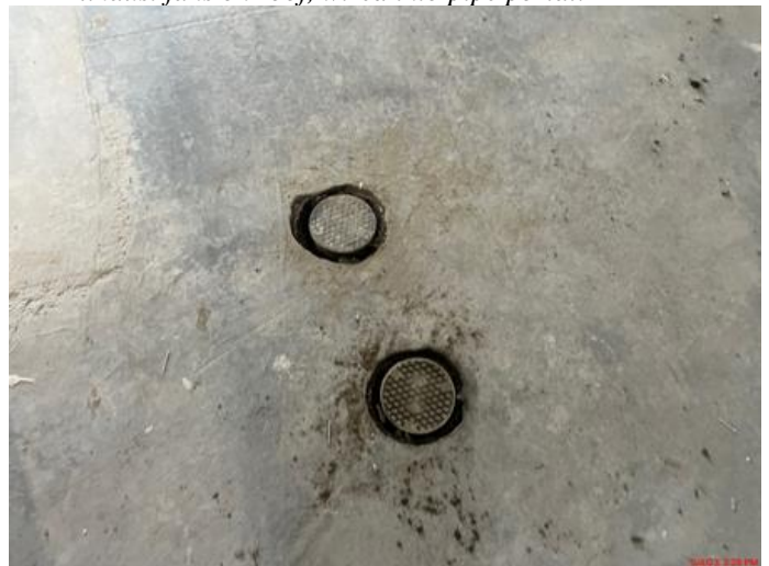
Drains exposed for epoxy installation Monday.
