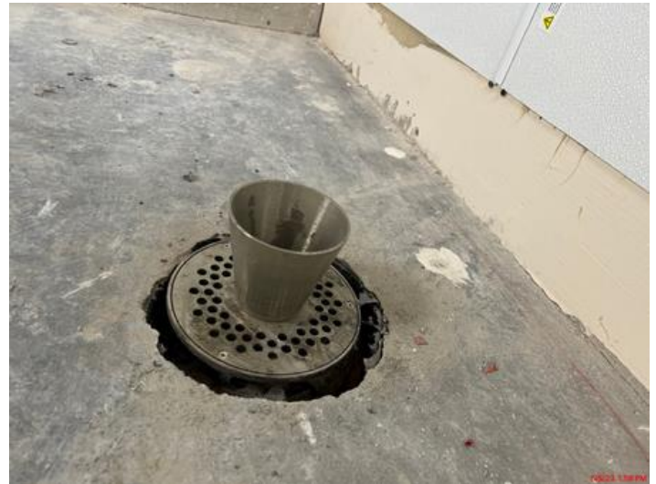
Funnel drain installed for epoxy installation.
