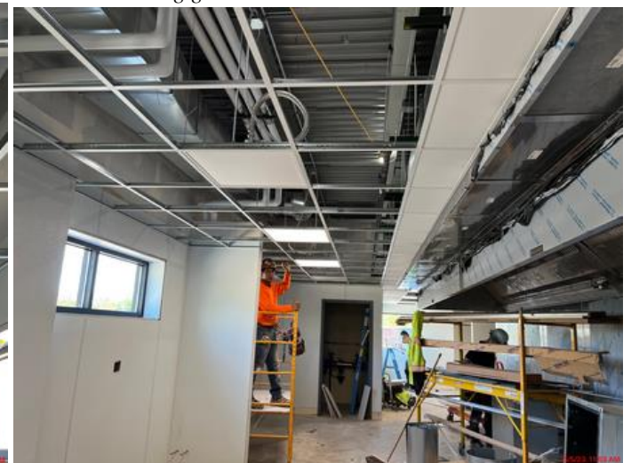
Ceiling grid with new lights installed.
