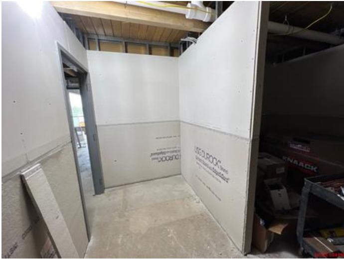
Durock and drywall installed in restrooms.
