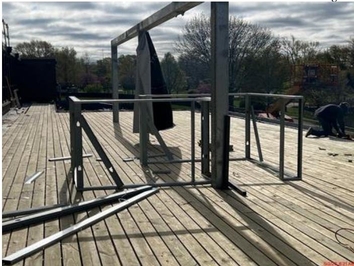
Server station framed up.
