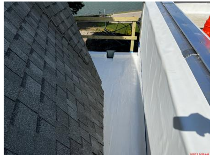
TPO installed from new roof to old roof.
