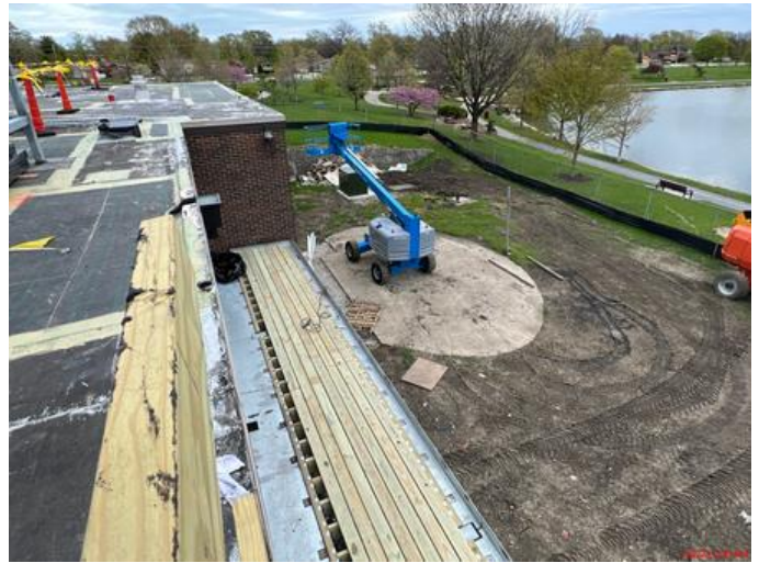
Decking being installed.
