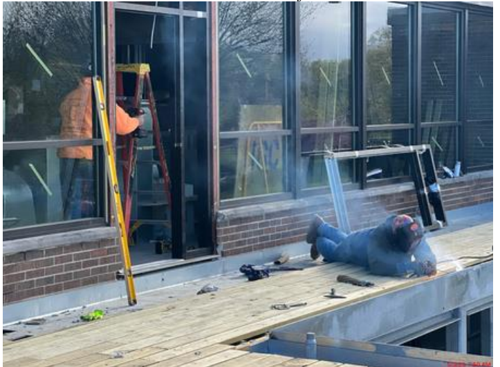
Closure steel plate being installed.
