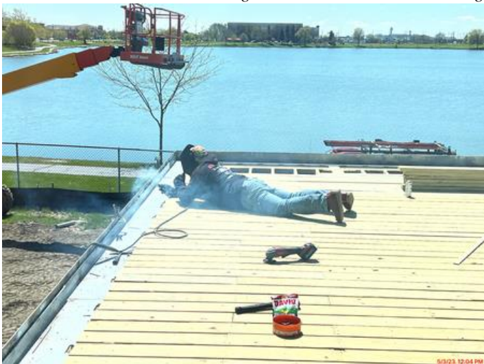
Closure steel plate being installed.
