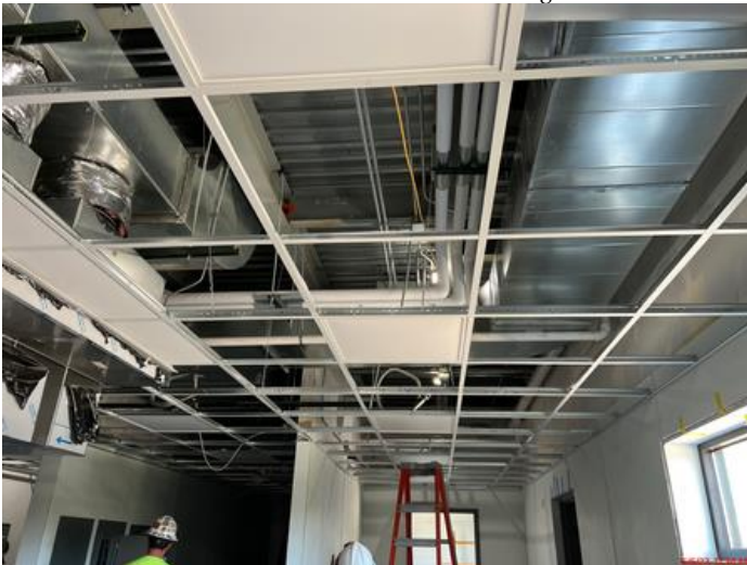
Ceiling grid with new lights installed.
