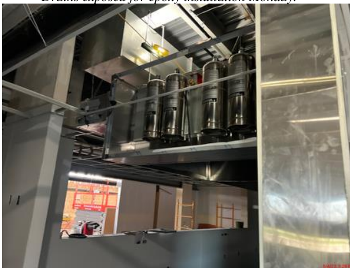
Ceiling grid being installed over door of Ansul system.
