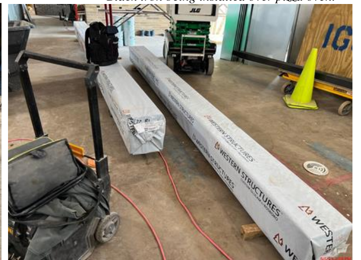
Mezzanine beams to be installed.
