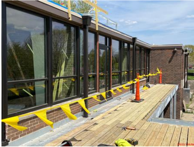
Gutters, new windows, and doors installed.
