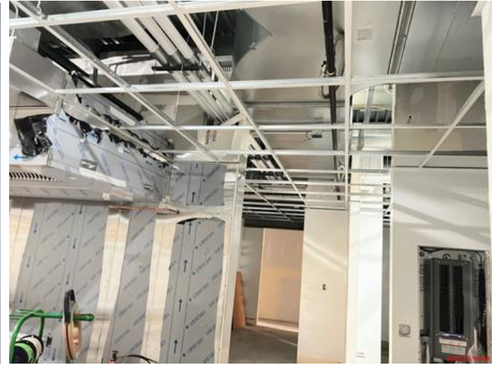
Ceiling grid installed.
