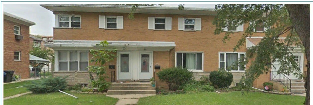
Figure 15. Typical building within Repetitive Loss Area 5. As shown above, many of the buildings in this area have extended their downspouts and sump pump discharges to drain away from the building.
