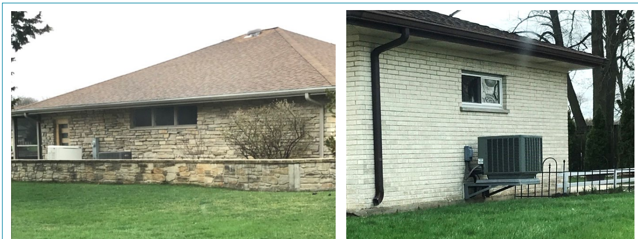
Figure 21. Elevated AC unit and private floodwall within Repetitive Loss Area 8
