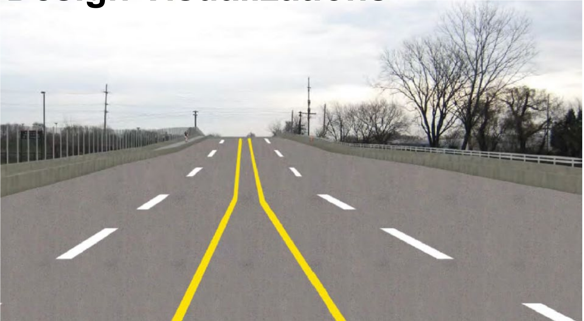
Looking east at Bridge over Union Pacific Railroad
