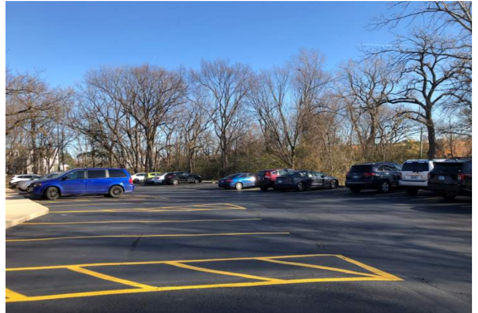
View of parking lot facing east
