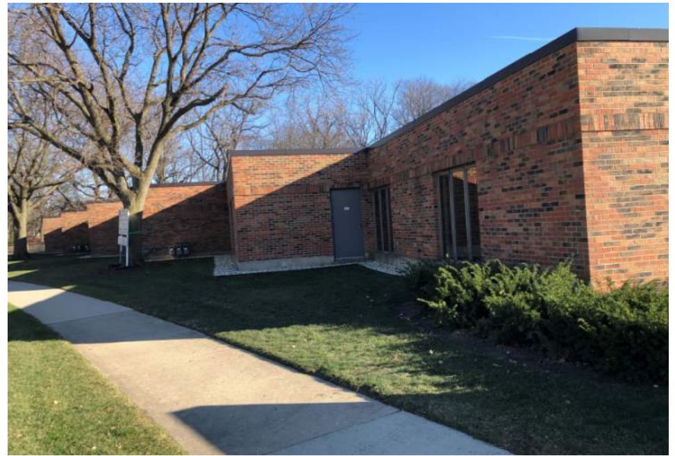
North side of office building, facing Elk Blvd
