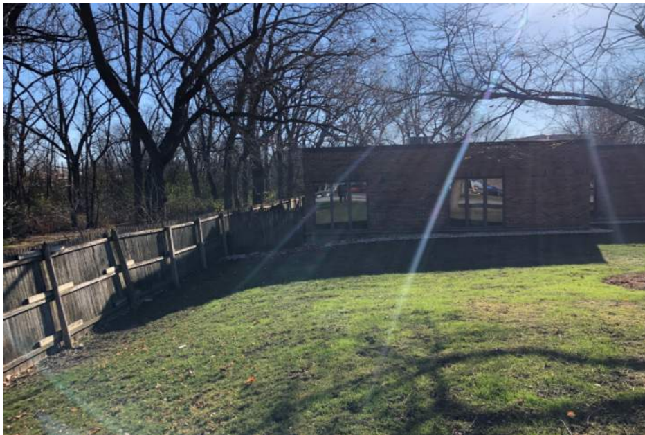
View of separation between residential property to the east and office complex; separated by six foot tall, solid fence
