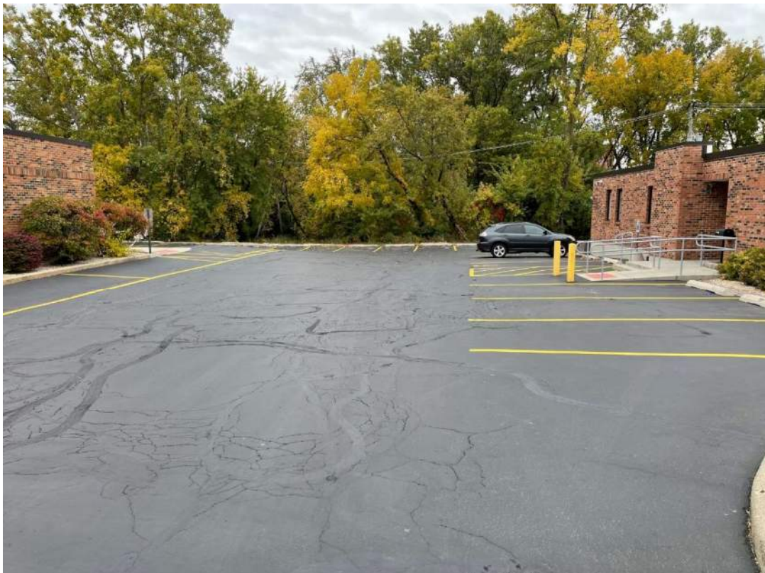
10. View of parking lot near the entrance of the office complex.
