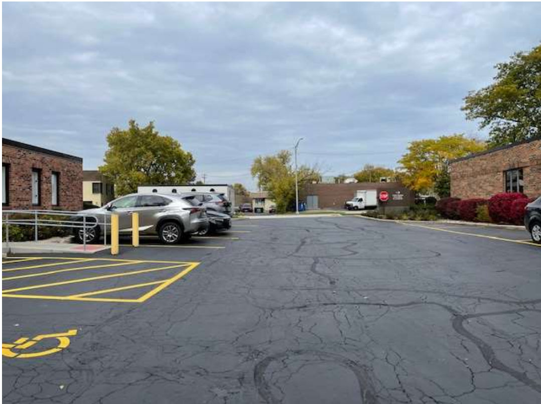
6. View of Handicapped parking space
