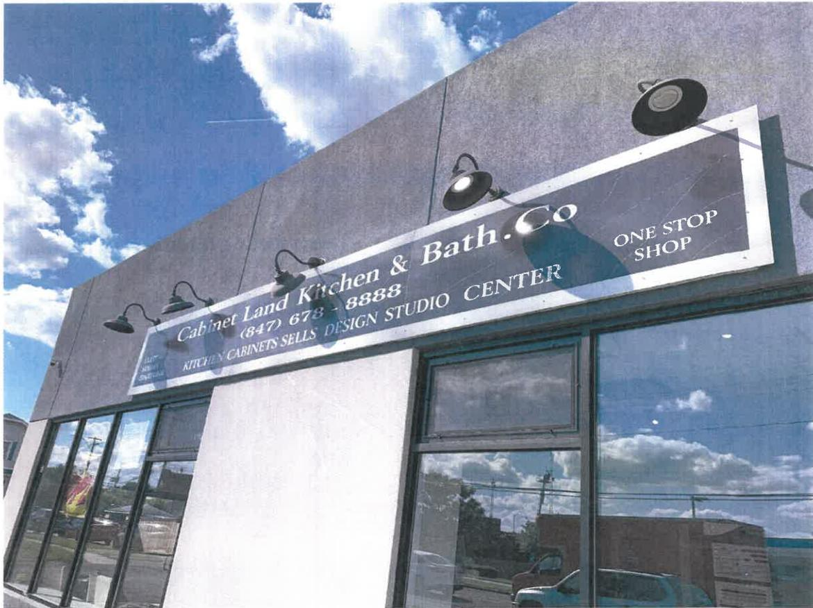
EXISTING WOOD FRAME IS TIED INTO THE WALL WITH 3/4" (THICK) AND 8' (LONG) KWIK BOLT LONG THREAD CARBON STEEL EXPANSION ANCHORS.
