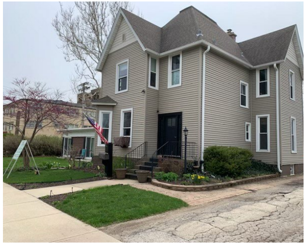
House, front (north) and side (west) elevations
