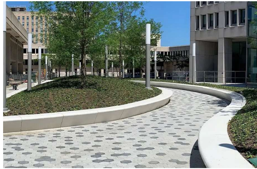
CAST IN PLACE CONCRETE SEAT WALLS
