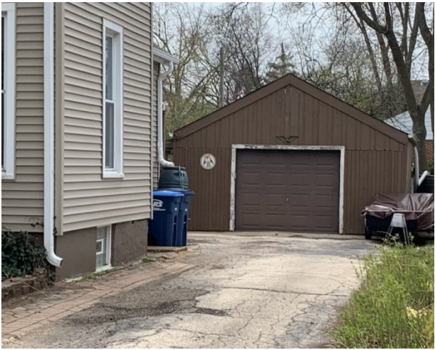
Existing detached garage
