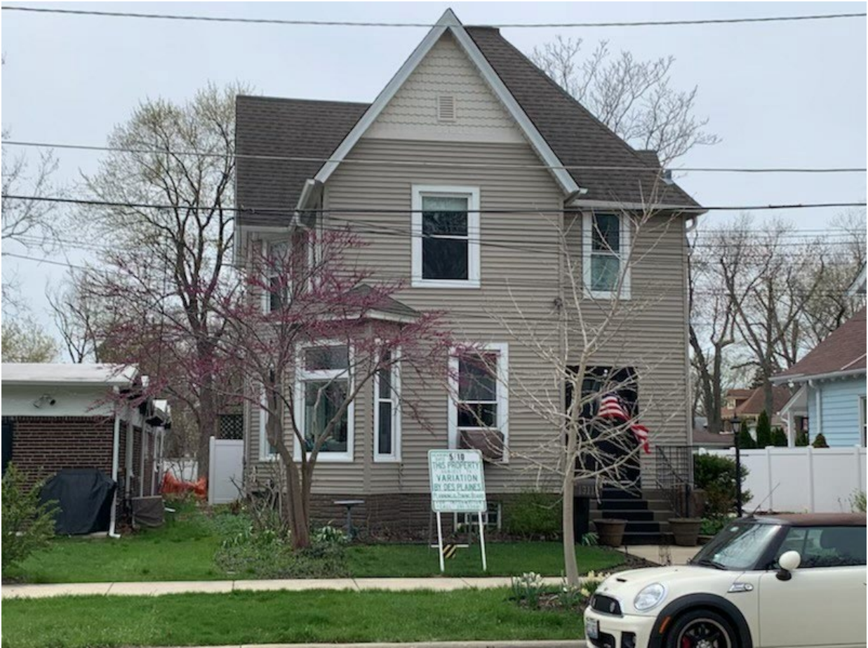
House, front (north) elevation
