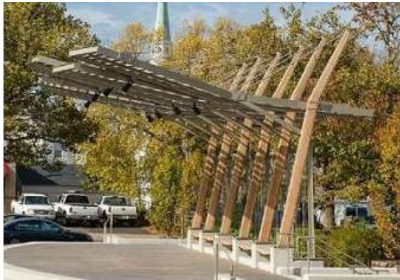
SHADE STRUCTURE ON RAISED PLATFORM
